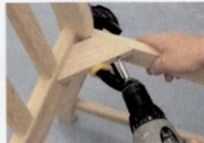
Glue and screw back corner blocks
